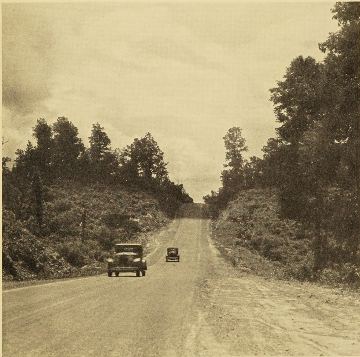
BITUMINOUS MACADAM SURFACING ON A SECTION OF US 60 IN WEST VIRGINIA
